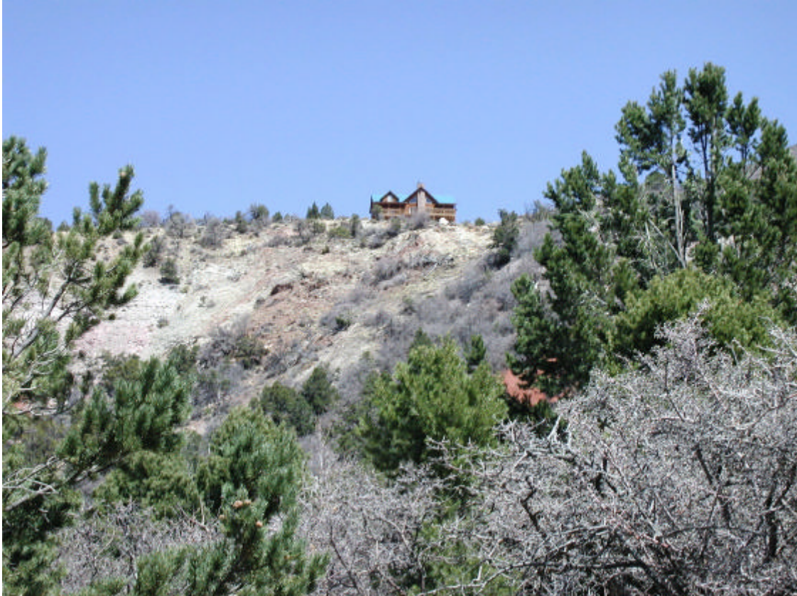
Home threatened by a small landslide that has formed on the headwall scarp of the much larger Green Hollow landslide near Cedar City, Utah.
