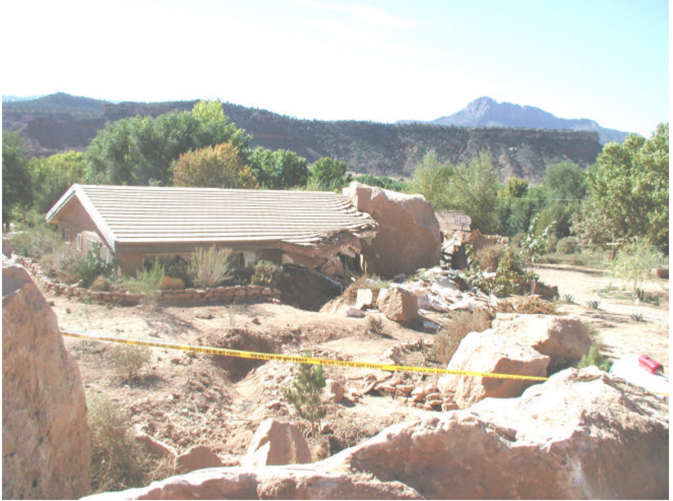
Home destroyed by a rock fall on October 18, 2001 in Rockville, Utah near Zion National Park
