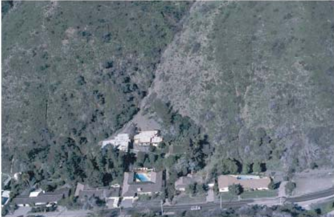
Figure 16 Debris flow deposited on small alluvial fan, Santa Monica Mountains, Los Angeles County, 1980, damaged the two houses built on the apex of the fan.
