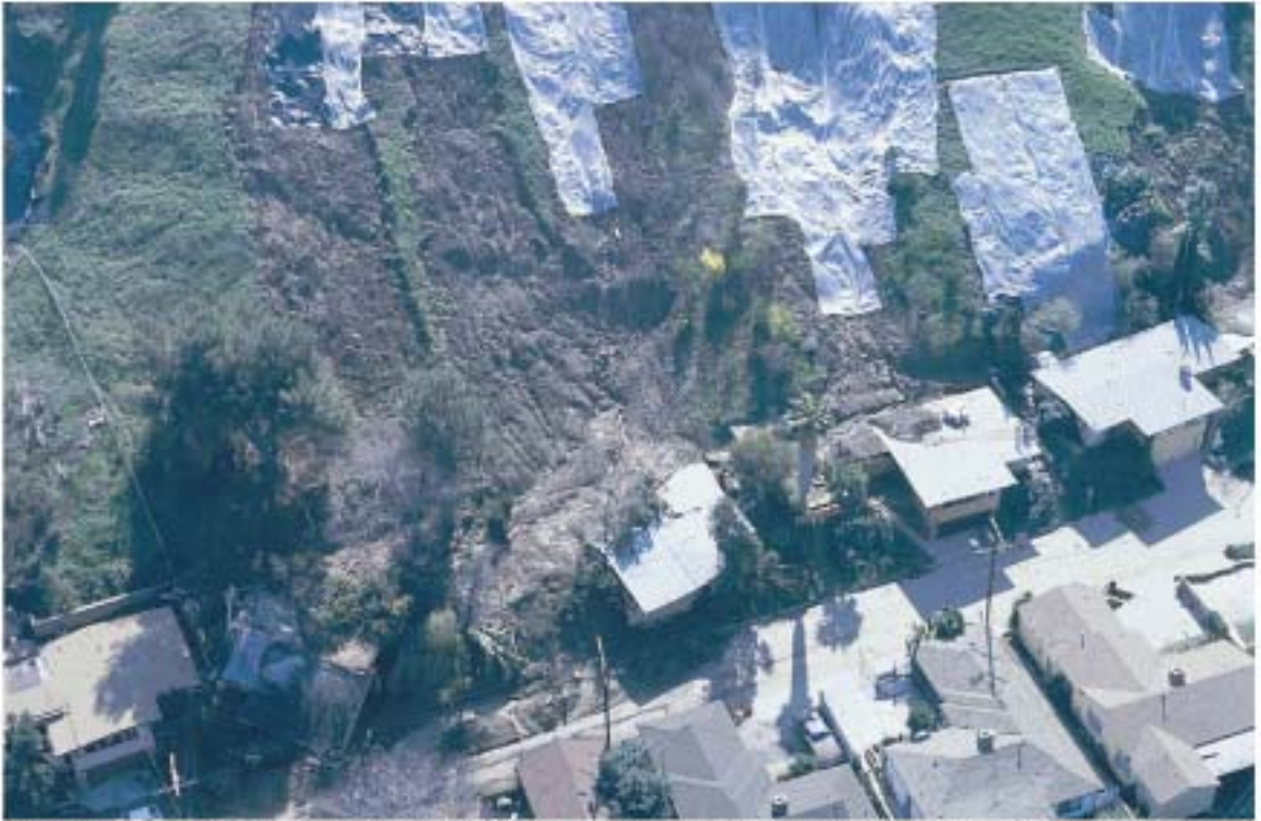
Figure 3 Multiple debris flows, Repetto Hills area, Los Angeles County, 1980. Debris flows are in Pleistocene alluvial deposits. Plastic sheets cover the upper parts of the debris flows.
