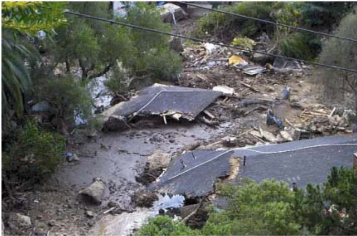
Figure 17 Structural damage produced by debris flows, Laguna Canyon, Orange County, 1998.
