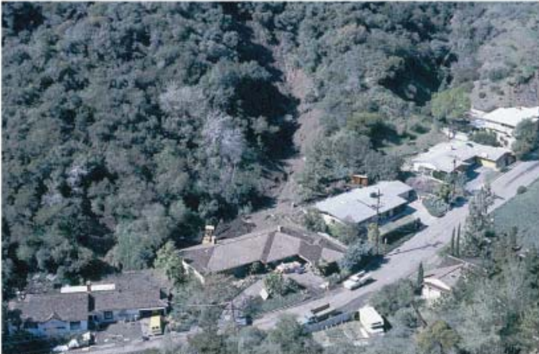
Figure 15 Debris flow deposited on small alluvial fan, Santa Monica Mountains, Los Angeles County, 1980. Brown roofed house near center built on a small alluvial fan was damaged by a relatively small debris flow.
