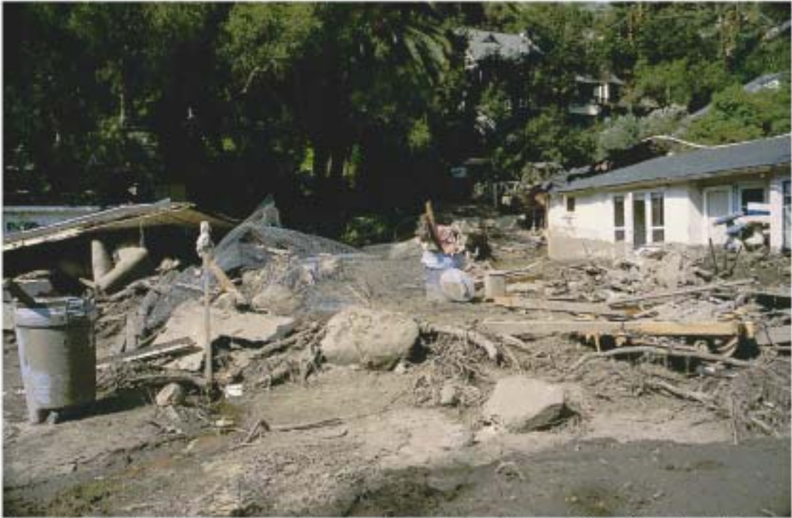
Figure 18 Structural damage produced by debris flows, Laguna Canyon, Orange County, 1998.
